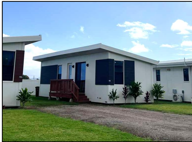
Temporary housing units adjacent to the Housing for Healthcare Initiative
