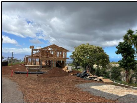
Kula Rebuild: February 2026
